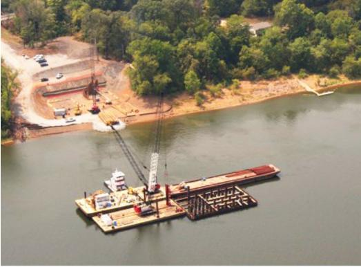
The use of the "follower" enabled Mahan to install the pile more efficiently since it cut down on the amount of labor and materials necessary to install these large casings. C.J. Mahan prides itself on finding innovative solutions in heavy foundation construction for the benefit of the owner.
