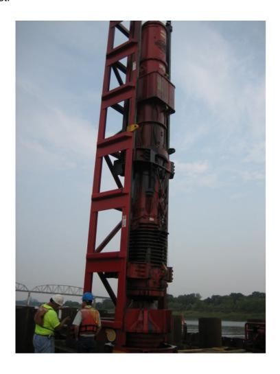
Since the final cut-off elevation of the pile was 39 feet below normal pool, there would have to be a third extension welded to each pile in order to drive them to the required tip elevation. This extension was added to two of the piles, so the hammer could be tested, but Mahan took another approach to driving the remaining pile.
