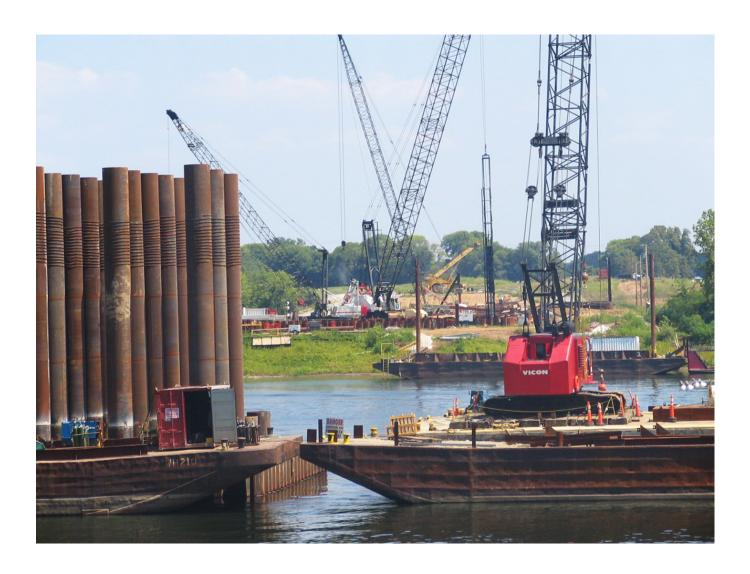
A vibratory hammer was used to penetrate each pile approximately 75' into the river bottom. The final penetration was achieved through the use of a Pileco D125-3 single-acting diesel hammer, which is made for offshore applications and had never been used in the Midwest.
