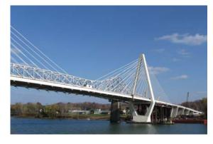
The post-tensioned concrete bridge deck was cast in segments. Each segment was constructed completely on form travelers that were suspended from the bridge deck. Once a segment was poured and cured, the form travelers were advanced to make preparation for the next pour. The main towers of this bridge, which rise 250 feet over the Ohio River, are founded on massive foundations
