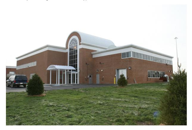
This project consists of an entirely new 39,150 square foot building which extends 77 feel below ground to house six huge Raw Sewage Pumps with GE motors and discharge piping capable of pumping over 330 million gallons of sewage per day.
