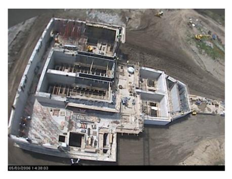
The facility also allows for future facilities that will allow up to 550 million gallons per day. Other major features on the Contract include a variety of complex mechanical processing systems, over 3000 feet of 104" Interconnector Sewer, over 600 feet on Castin-Place Box Culvert up to 18' x 14' in size, four round Cast-in-Place Junction Chambers ranging in size up to 56 feet in diameter and 50'-6" tall.
